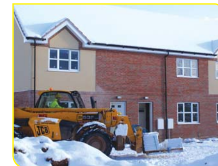
Work continues in the snow at Riseholme Rd, Gainsborough
